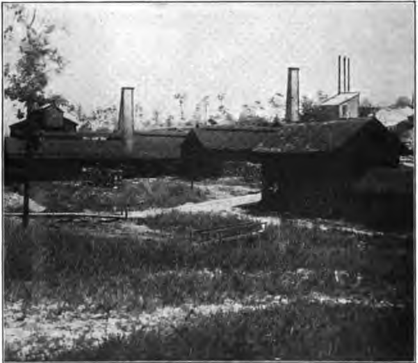
CHEMICAL REDUCTION PLANT—HAILE GOLD MINE.
